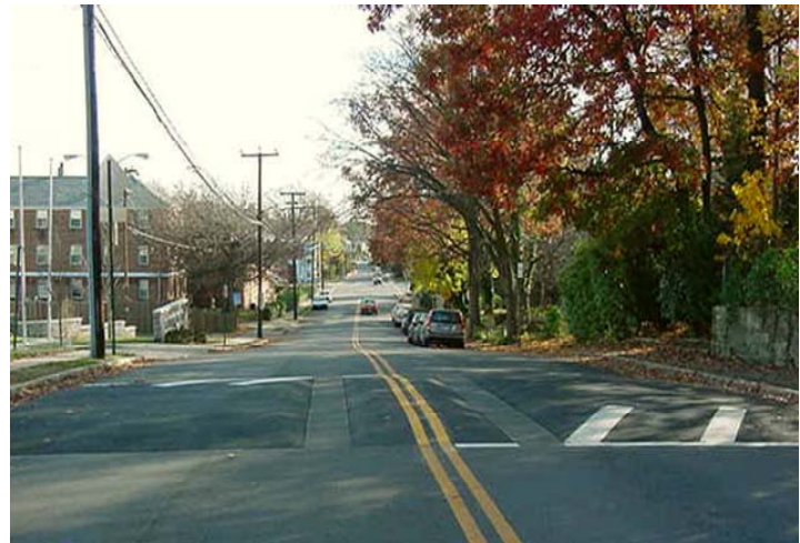
Speed Cushion – North Fillmore Street
